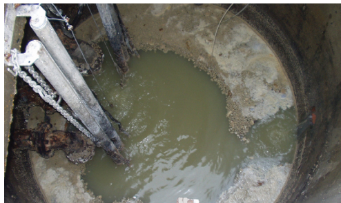
Clean-up: the bacteria system helps break down grease
